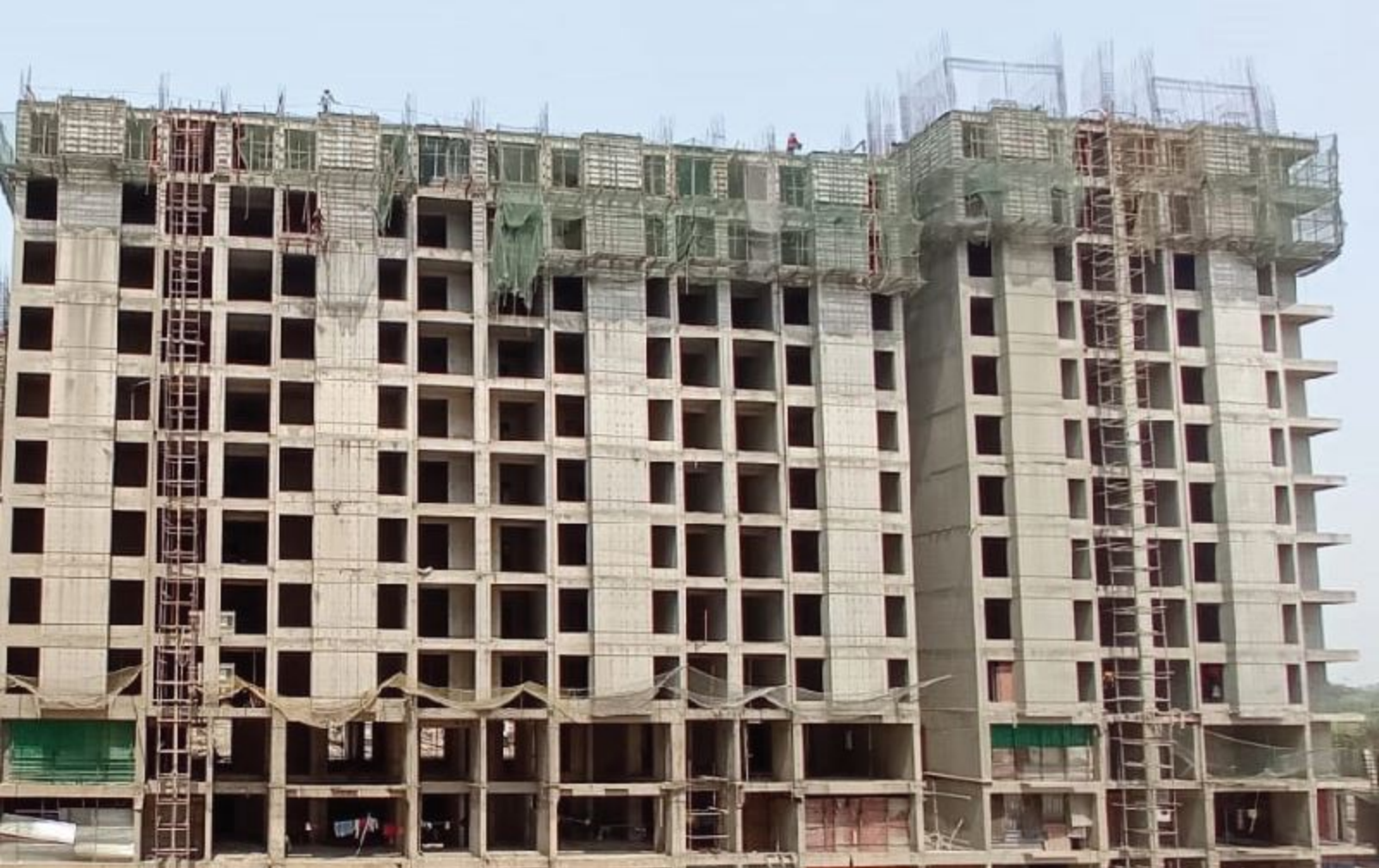
TOWER-6 (B):: Slab at 12th Floor Level Completed
